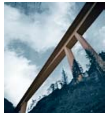
Schottwien valley bridge
