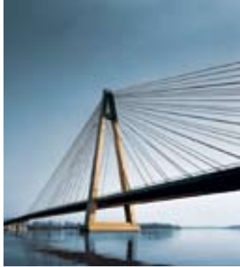
Danube bridge, Tulln
