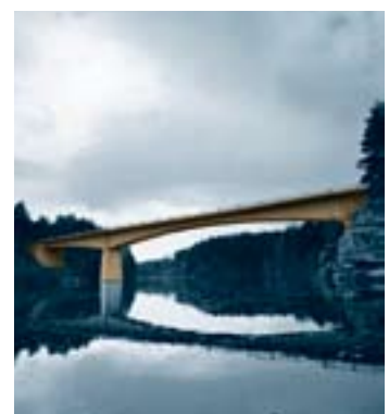
Ottenstein reservoir bridge
